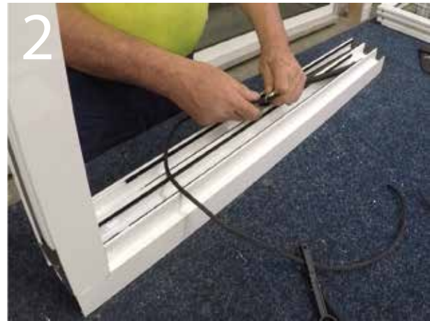
2. Replace spring plastic wrings with long cord or string for easier access
