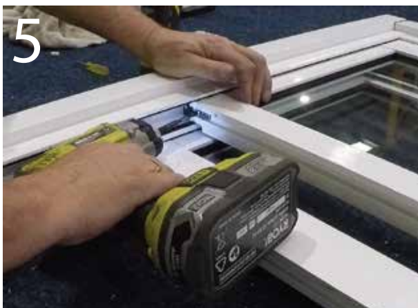
5. Screw/pop-rivet friction feet onto bottom of sash
